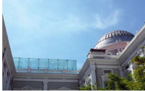
Exterior of Glass Passage Photo: ©Arup / Kelvin Kan
